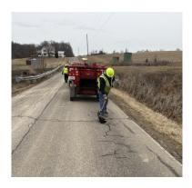
In 2024 we scheduled to repair roads and responded to travelers calling in about potholes with cold patch and hotmix. We worked 350 hours total over the year placing cold patch for a cost of \$90,782.20 material and \$11,209.82 labor. We also repaired with our durapatch hot mix for a cost of \$34,439.80 material and \$13,798.83 labor.
