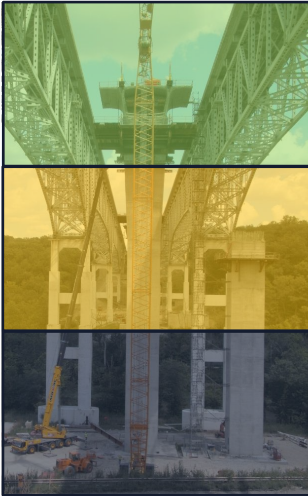
Multiple concrete placement procedure
