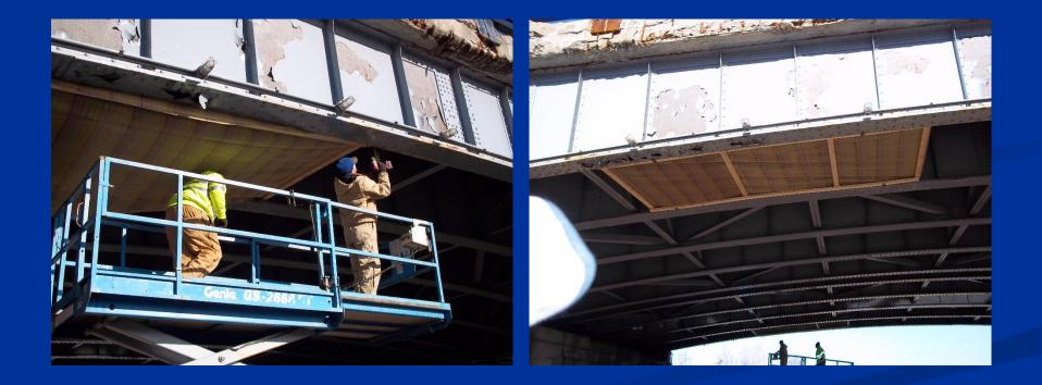
Used perforated tarp on end sections to allow drainage to flow thru from the scuppers
