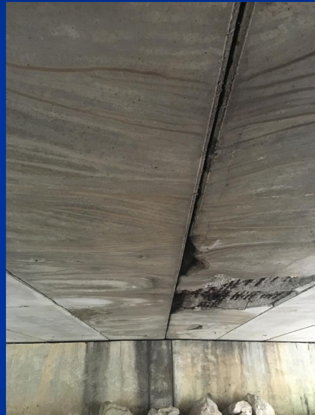
Staining on other center beam
