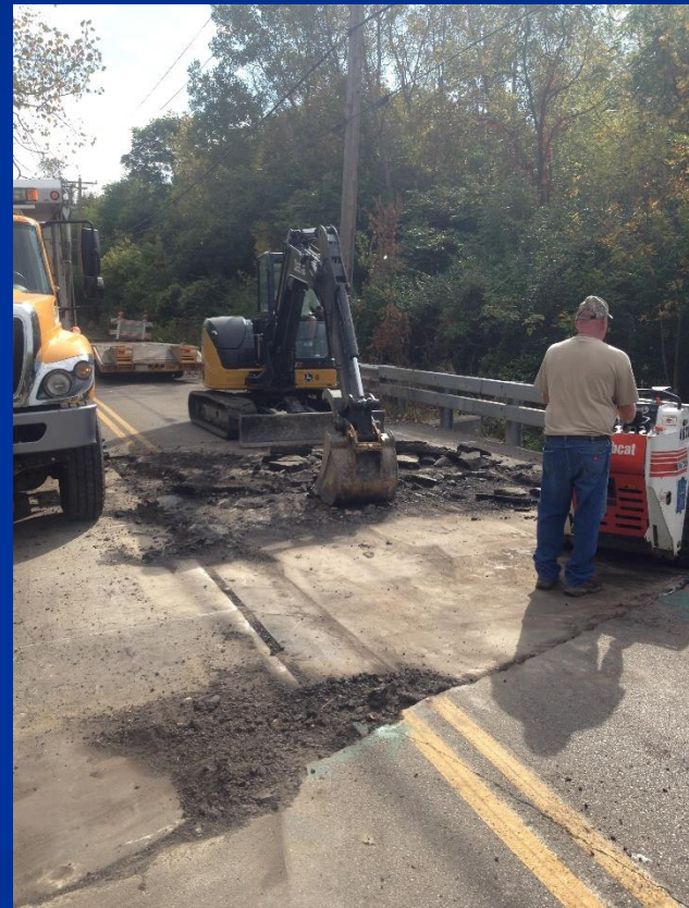
Removing asphalt
